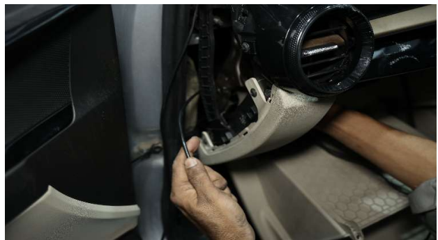
STEP 76 :- BRING CABLE NEAR THE GLOVEBOX AREA FOR NEXT CONNECTIONS.
