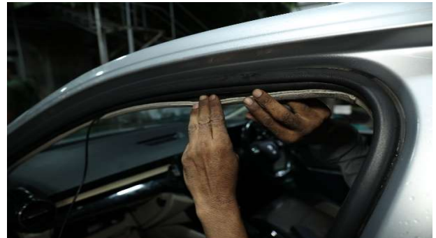
STEP 72 :- ROUTING CABLE THROUGH THE ROOF LINER FROM B-PILLAR TO A-PILLAR.
