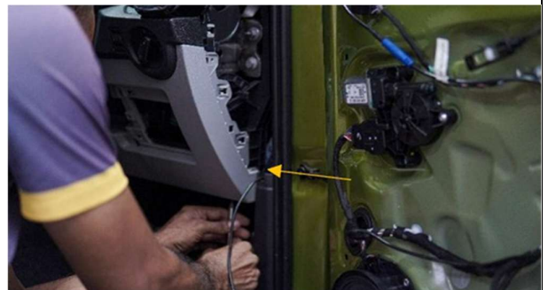
STEP 53 :- REPEAT THE SAME PROCESS ON THE RIGHT DOOR, ROUTE EXTENTION CABLE AS MARKED.
