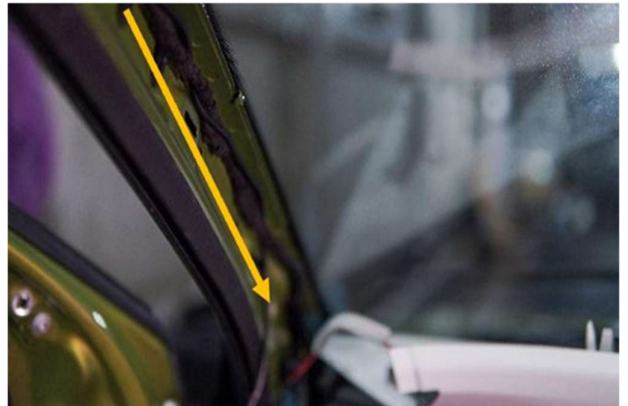
STEP 74 :- ROUTE CABLE UNDERNEATH A-PILLAR.
